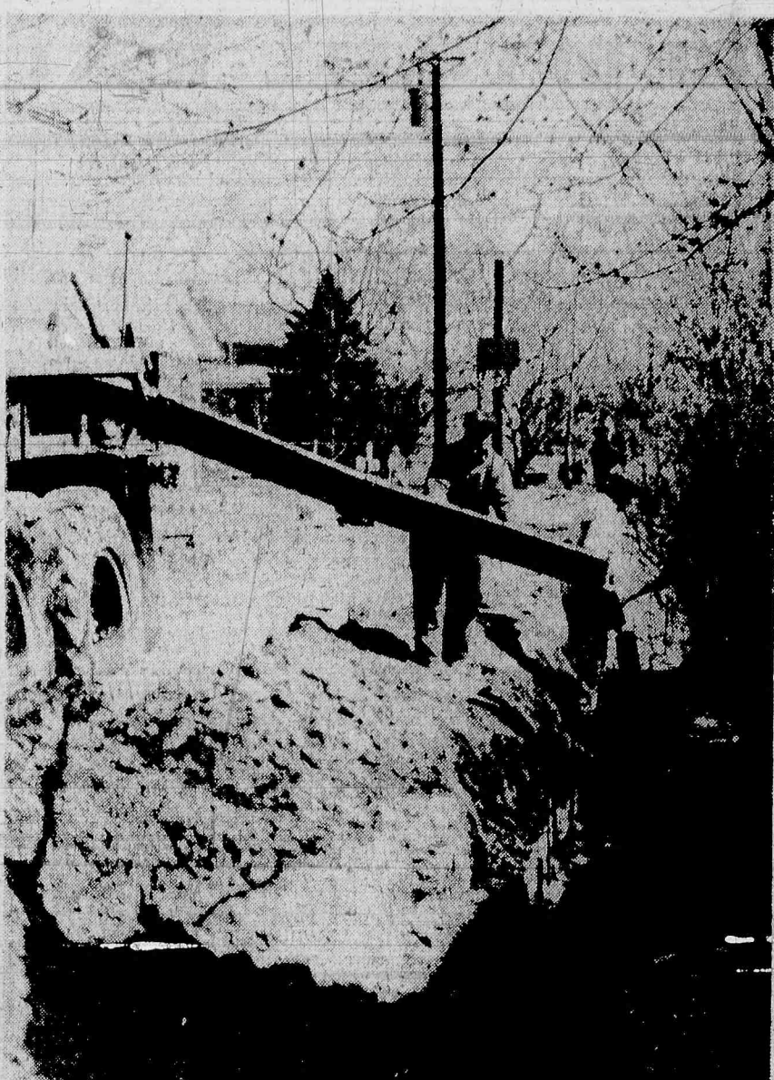
CURBS — Contractors pour wet cement from a truck into wooden molds to prepare curbs for Belleville's newest thoroughfare: Park Place. A second new street is scheduled for construction. That road will be Laurel Court.
